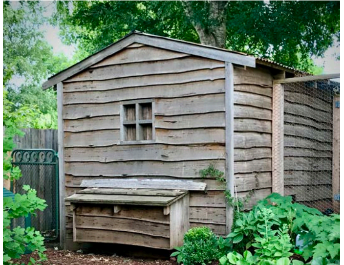
Country chook shed built with radially sawn timber
